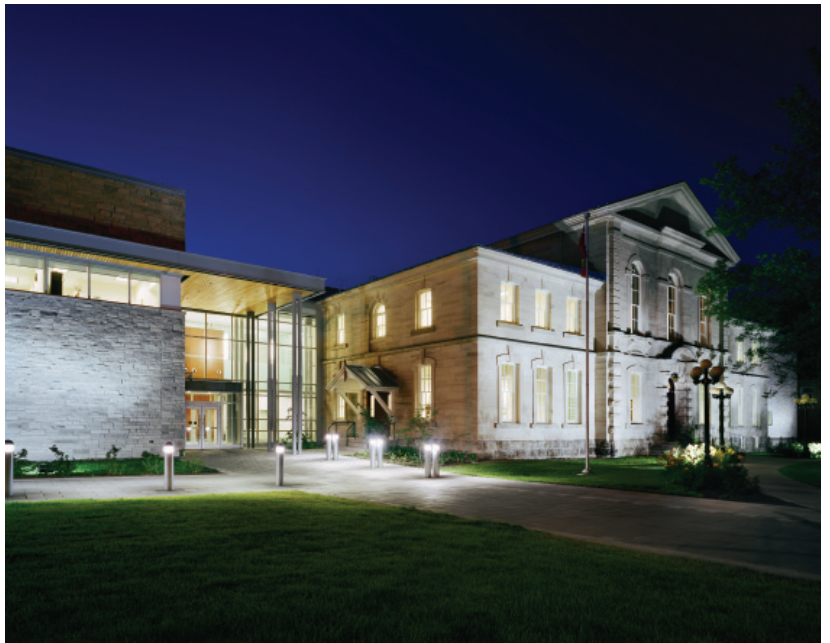
The New Renfrew County Courthouse
